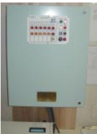
Alarm board attached to the wheel house wall (left) and hold sensor attached to the cargo hold (seen along the ladder)
