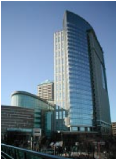
Universal's new office building
