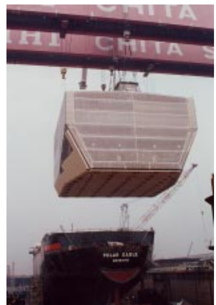
Appearance of IHI SPB tank
