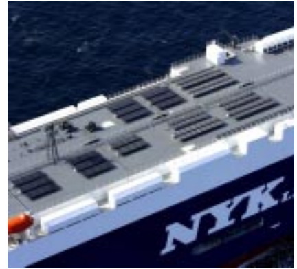
40kW solar photovoltaic system arrangement on the garage top deck
